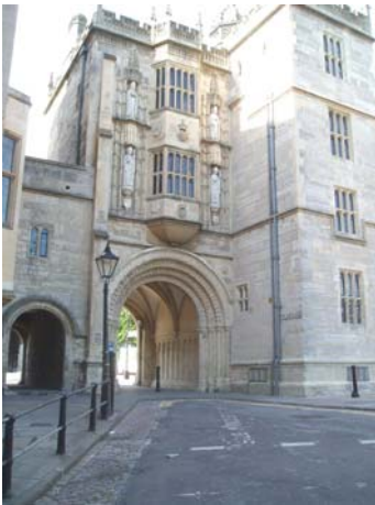
Refurbished Norman Arches, Bristol Cathedral
